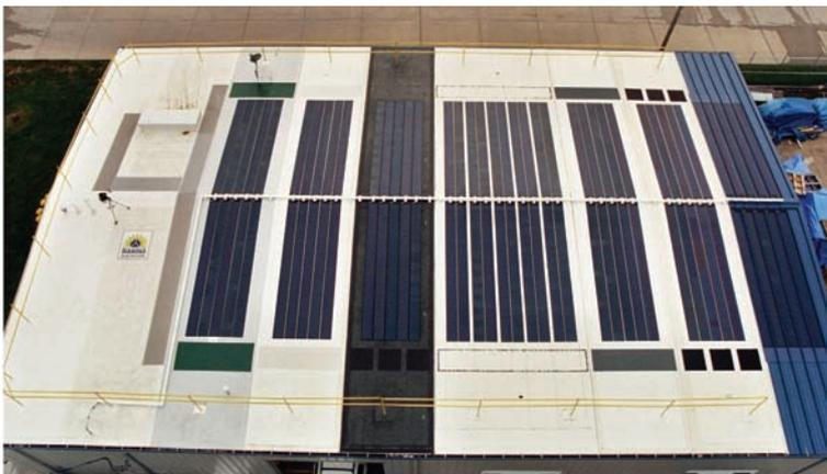
**BIPV testbed** This PV demonstration project, which features seven different roof membranes, was installed at Diamond Roofing Company’s facility in Manhattan, KS, with support from the Midwest Roofing Contractors Association. To monitor how the addition of BIPV laminates affects roof membrane temperature, 32 thermocouples installed around and under the subarrays are being monitored over a 3-year period.
