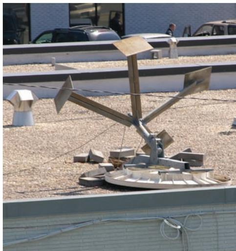
**Weathering the storm** As documented here by one of FEMA's Hurricane Charley and Katrina mitigation assessment teams, ballasted equipment is less likely than structurally attached equipment to remain stationary in the event of an extreme wind event.
